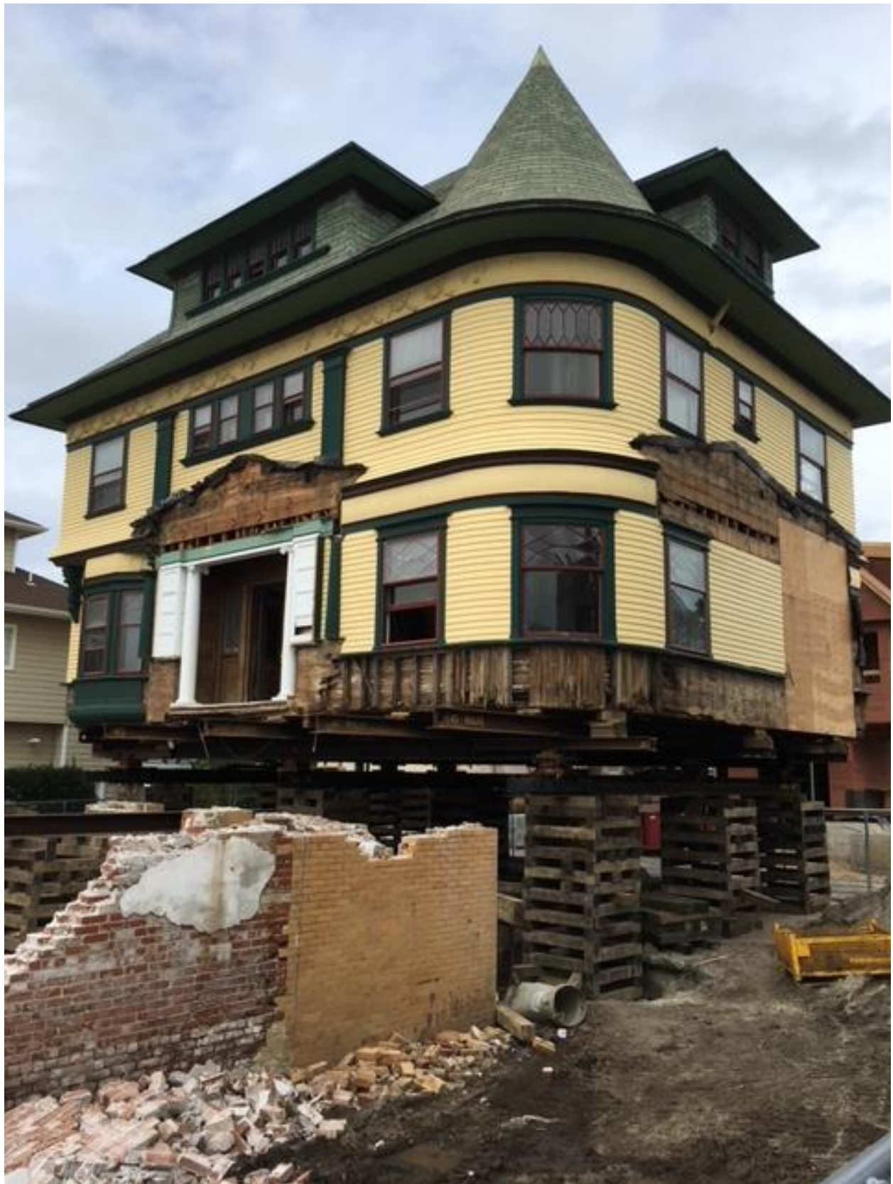
House during lift and relocation phase
