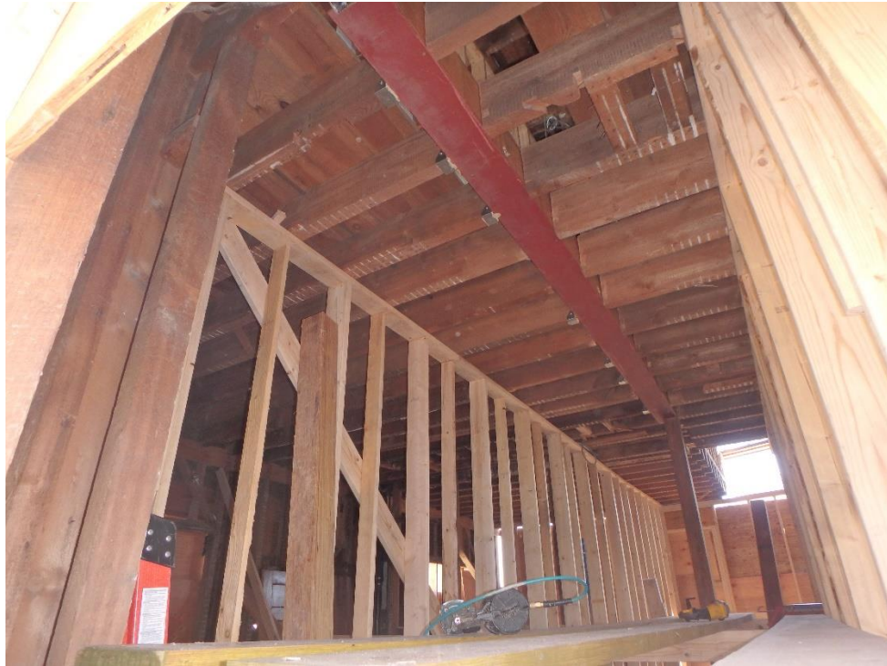
One of the new flush steel beams during construction
